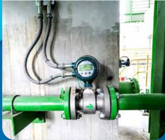
FLOW METER INSTALLATIONS
